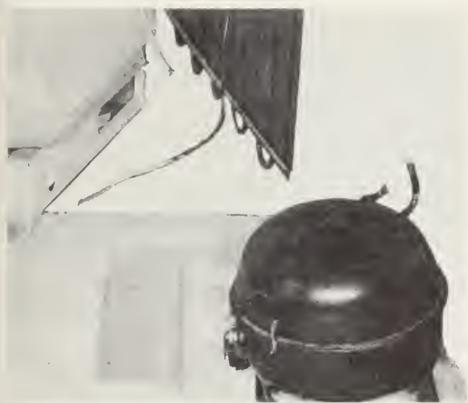
17-26. The old motor-compressor removed and its refrigerant lines sealed by pinching. This protects the internal structure of the unit for shipment. (Philco Corp.)
